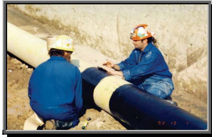
Figure 2-5. Visually Inspect Tape Wrap Installation. Remove Excess Wrinkling and Air Pockets. Recoat.
