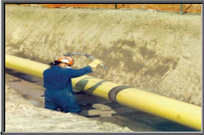
Figure 2-1. Remove Old Coating.
