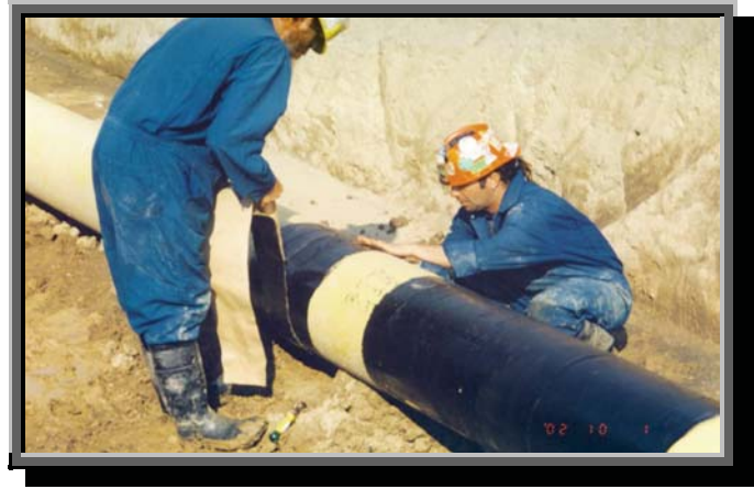
Figure 2-4. Let Primer Dry. Apply KEMA Series 60.
