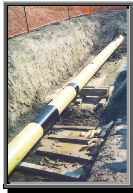
Figure 2-6. New Wrap is Ready for Spark Testing.
