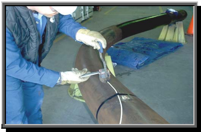
Figure 1-1. A trainee fastens a lead wire to a steel pipe with a thermite weld(er).
