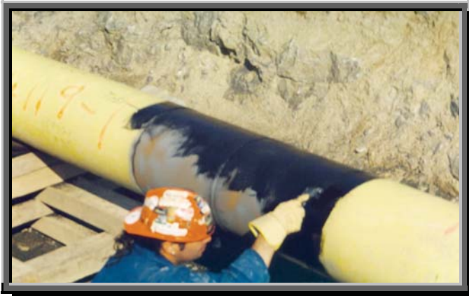
Figure 2-3. Apply Liquid Primer.
