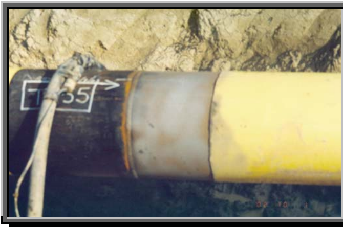
Figure 2-2. Minimum Power Tool Clean.
